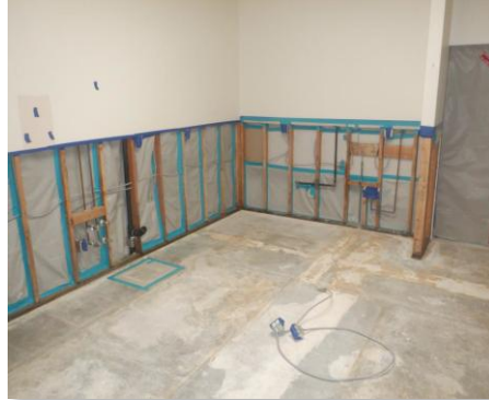
kitchen, looking towards sink
