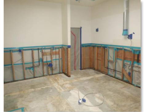
kitchen, looking towards oven
