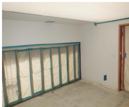
storage room, looking towards door and wall shared with kitchen
